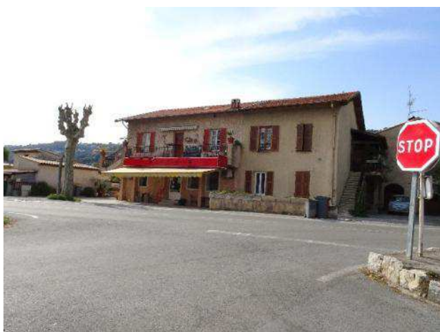
Figure 34 : Restaurant Les Frangins © Egis 2019
